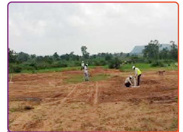
Completion of tower foundation work at North Karanpura-Chandwa (NKTL)
